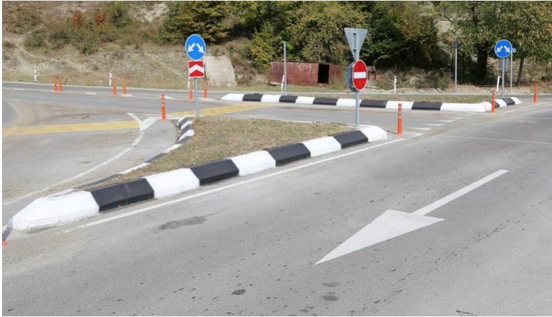
Road Narrowing through use of Islands in Georgia
